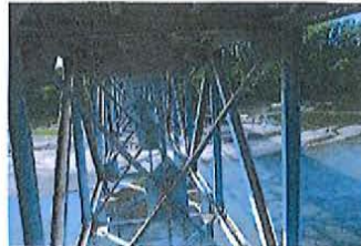
View of Truss Bridge
