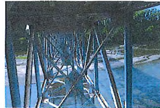
View of Truss Bracing
